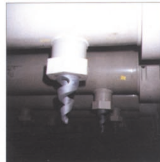
Helix full-cone nozzles in a flue gas cleaning plant
